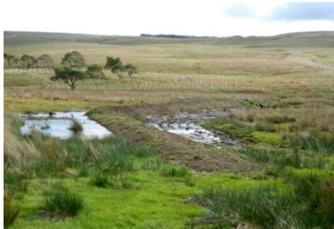
An Earth Bund on the Demonstration Site, designed to slow the flow of floodwater
